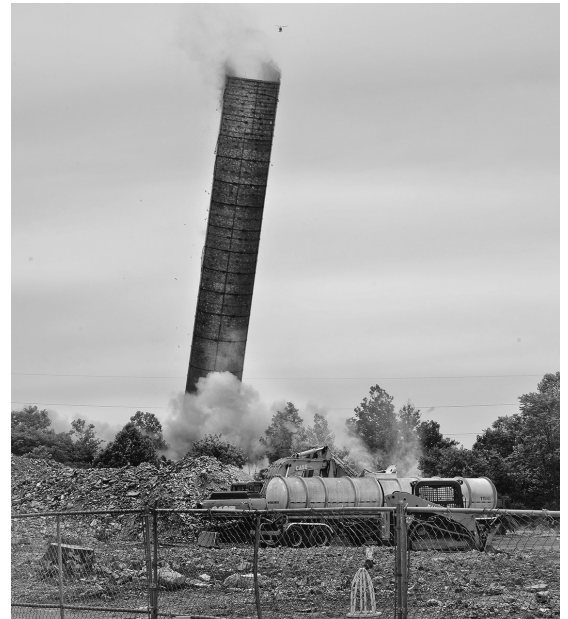
FMC fume stack being demolished. Photo credit Duke Realty, LP
